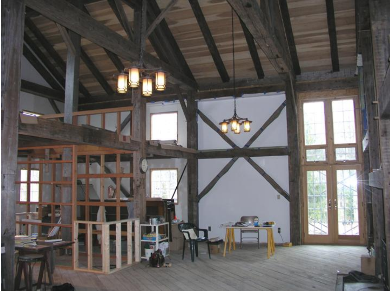
The interior of the Christian home with the framework intact from Methodist Church in Chenango Forks
