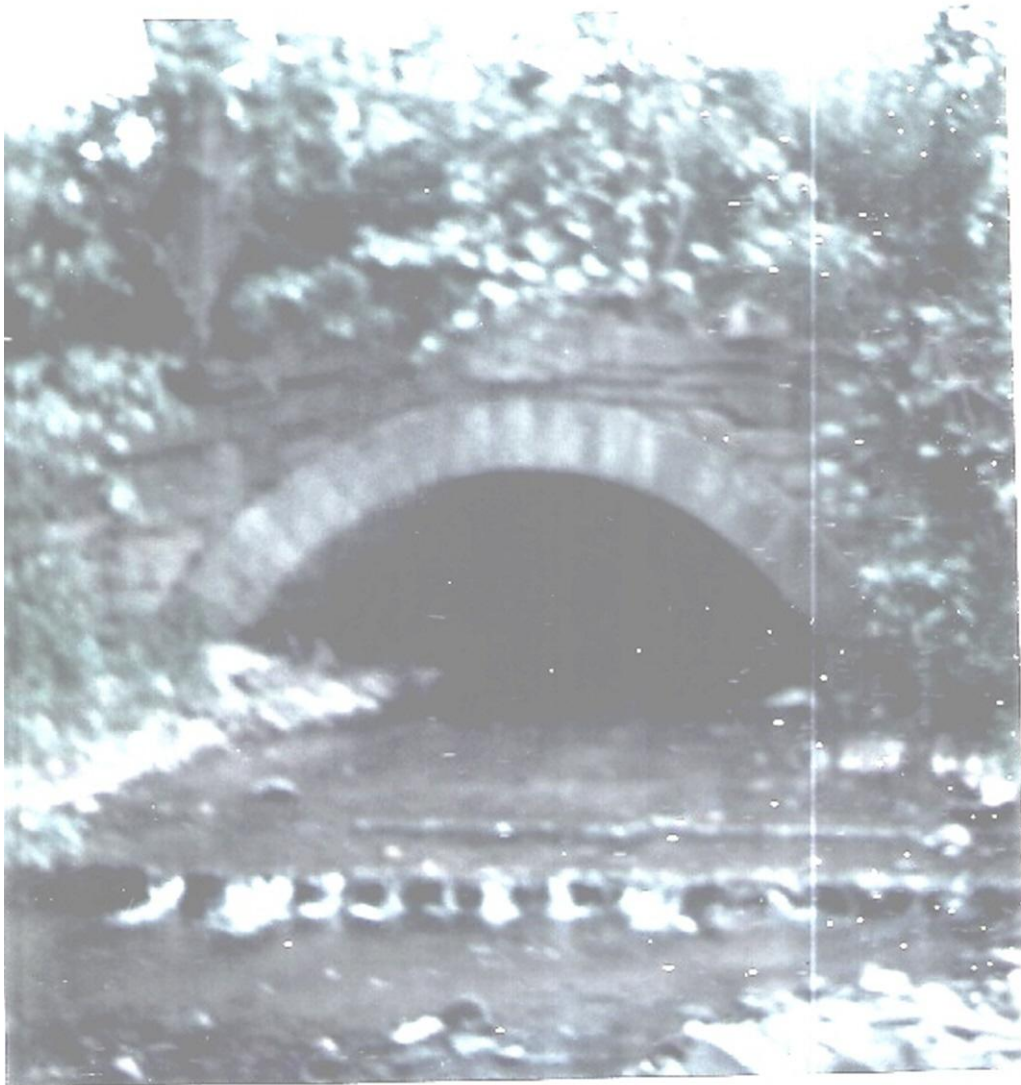
Stone Culvert under the Chenango Canal on Stillwater Road
